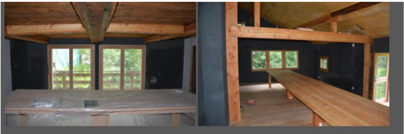
Figure ..... - Ithaka institute demonstrates biochar in practice as plaster on the walls
